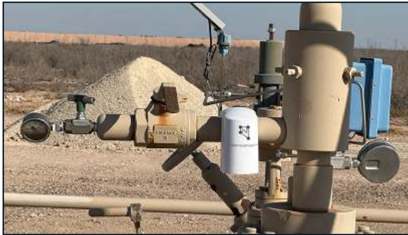
MethaneTrack™ wireless sensor mounted in close proximity to christmas tree well head
