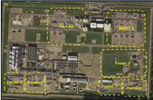
Installation of 155 wireless sensors in just 3 days
